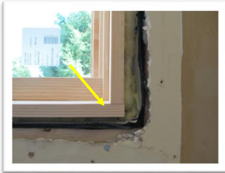
Frame in rough window opening
