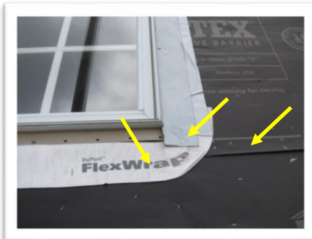
Building paper shingle wrapped – top layer over lower layer
