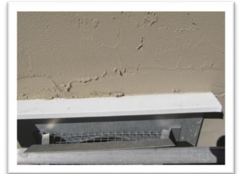
Fire flue is properly flashed
