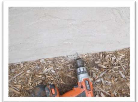
Wood below grade
