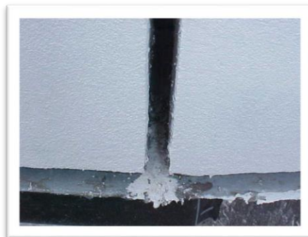
Expansion joint before caulk is applied
