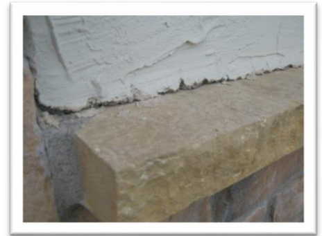
Ledge is sloped, not flashed or caulked
