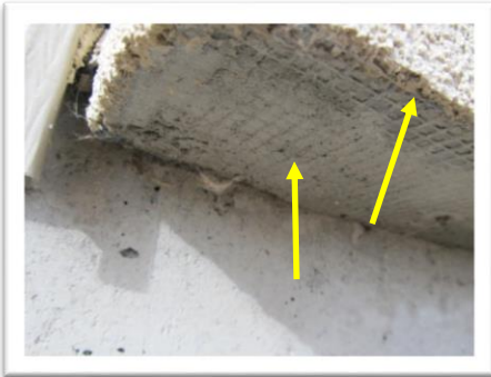
EIFS- 1/8" thick stucco with fiberglass mesh.
