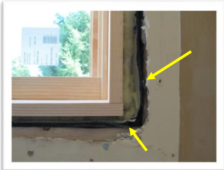
Rough opening window sill flashing
