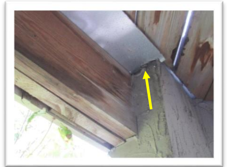
Deck column flashing
