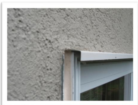
Window head flashing
