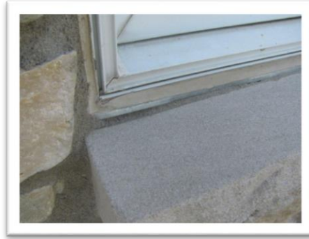
Good caulk joint
