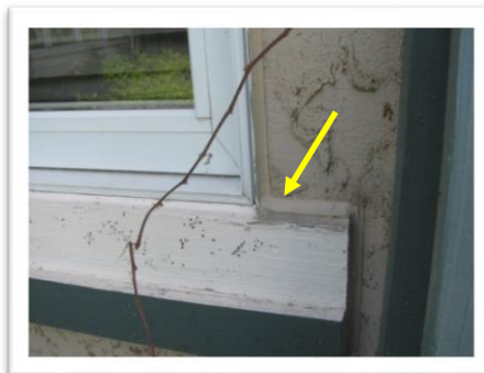
Good caulk joint
