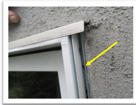
Stop bead provides a gap for a proper caulk joint.
