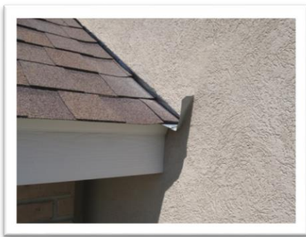
Proper kickout flashing
