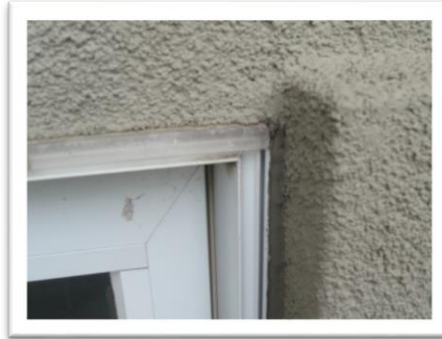
Drip flashing at window
