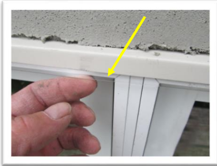
Drip flashing under head flashing of window
