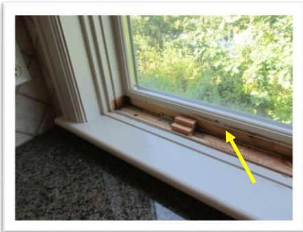
Fixed window sash
