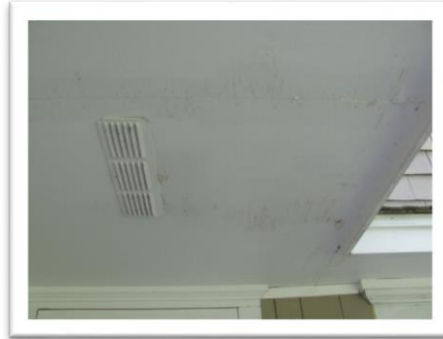
Large soffit overhang.
