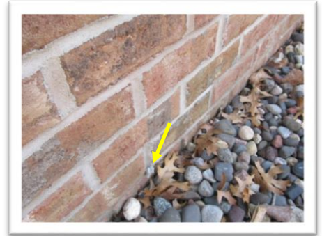
Weep rope in brick application
