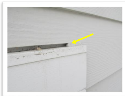
Caulk joint end dam
