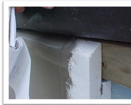
EIFS basecoat with mesh embedded over ESP foam board
