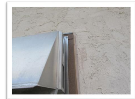
Vent is flashed and caulked
