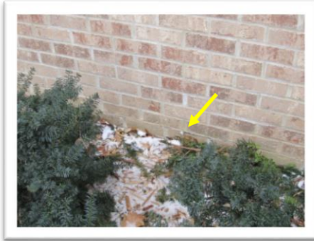
Weep rope in brick application
