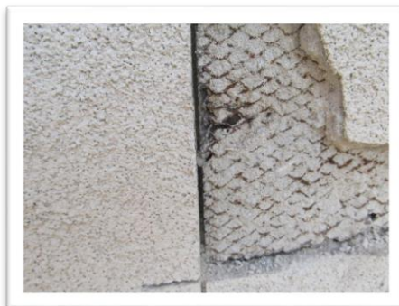
Metal lathe embedded in stucco
